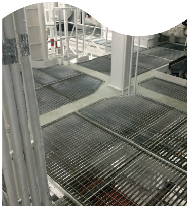
Mounting electrical carpentry, firefighting
