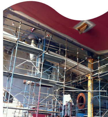
Planking, bridge and structure alignment
