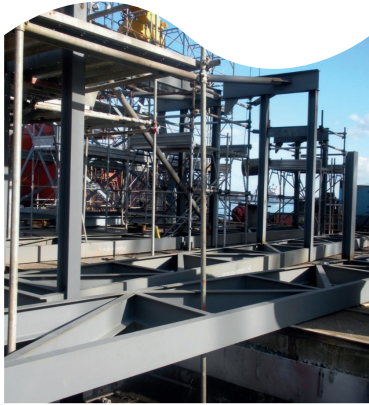
Pre-fabrication and pre-assembly activities
